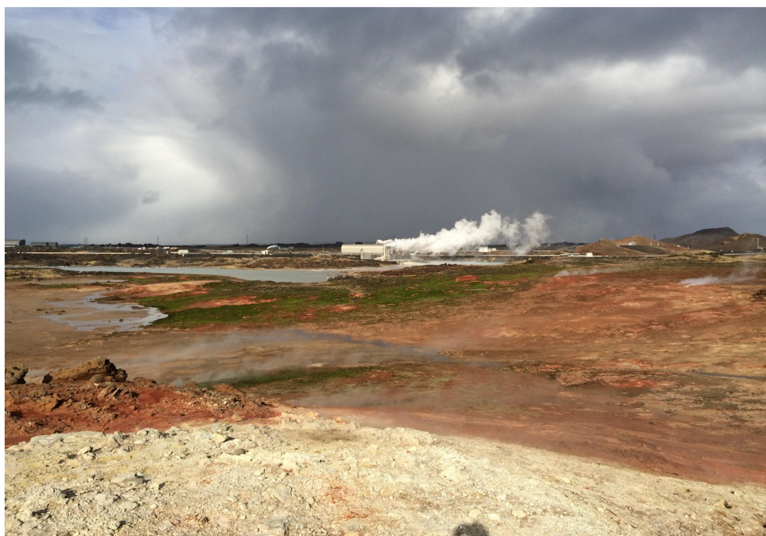
Figure 1 Reykjanes Geothermal Power Plant
